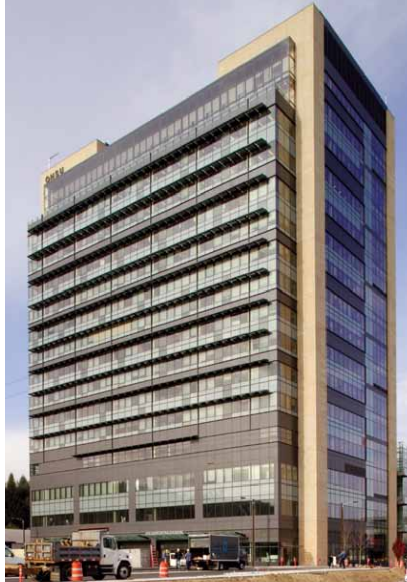
Five C60 ICHP microturbines used in a CHP application have reduced energy costs at this center for health and healing.
