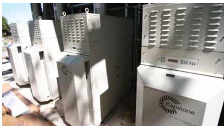
The pool at Foothill College is heated by four C60kW Capstone ICHP microturbines.
