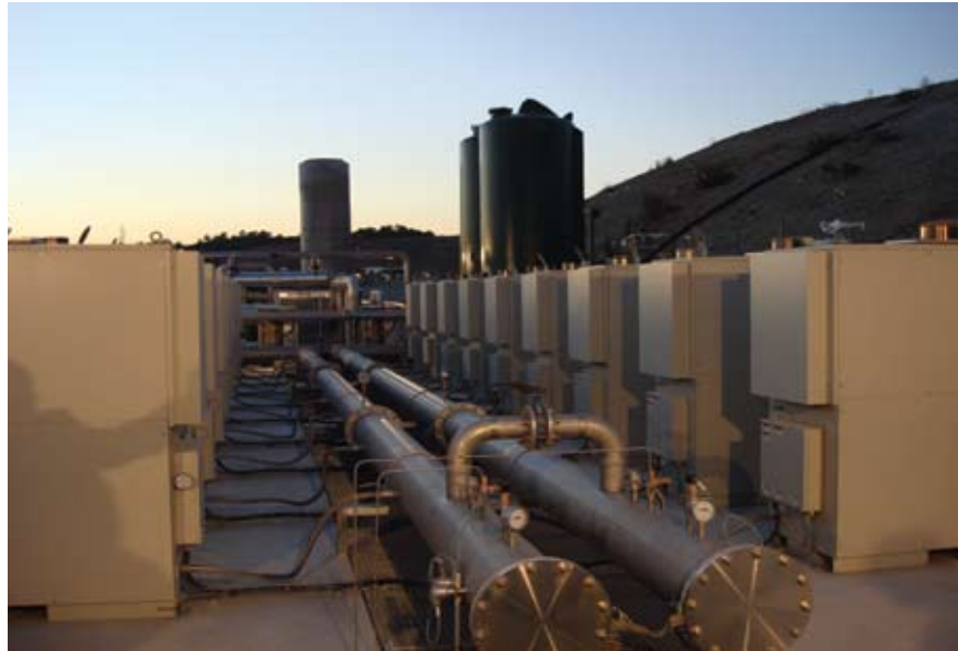
Eighteen C65 microturbines running on methane gas generate power and heat at Mentaure Landfill in France.
