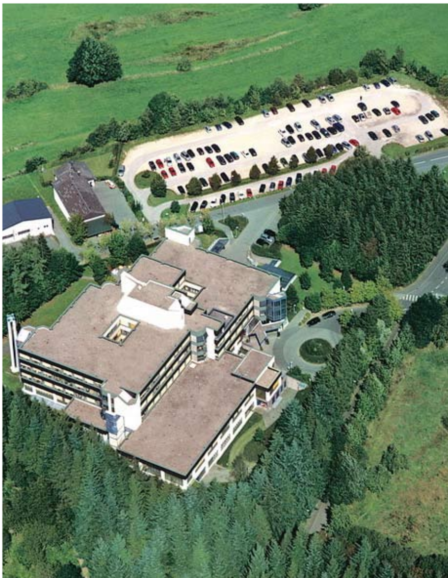
A Capstone C65 microturbine produces electrical and thermal power at St. Joseph Hospital in Germany.
