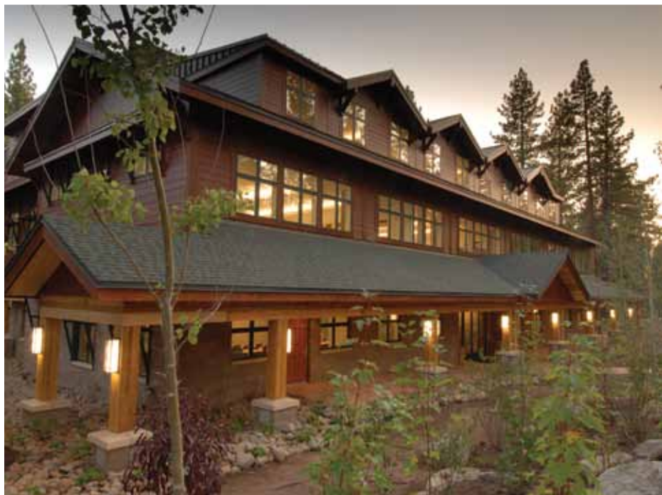
A Capstone C30 microturbine helps the Tahoe Center for Environmental Studies in California achieve LEED certification.
